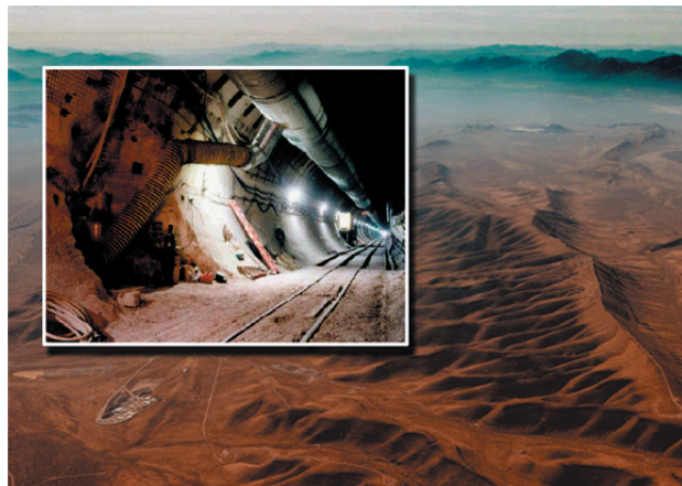
Yucca Mountain, located in Nevada northeast of Las Vegas, is the site of a permanent underground repository for high-level radioactive waste.
